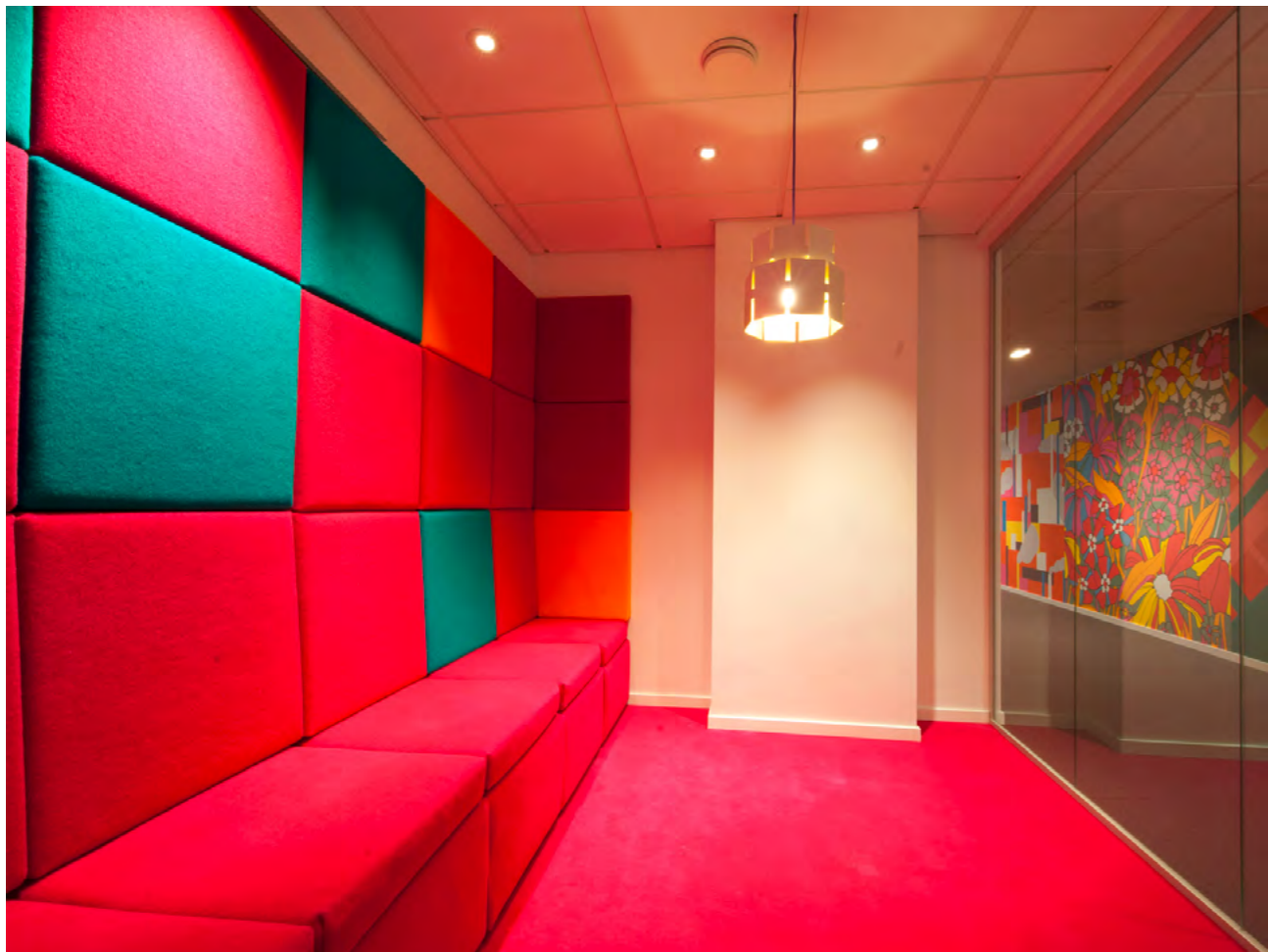
Particolare dei pannelli fonoassorbenti ricoperti in feltro. A detail of the sound-absorbing panels covered in felt.
